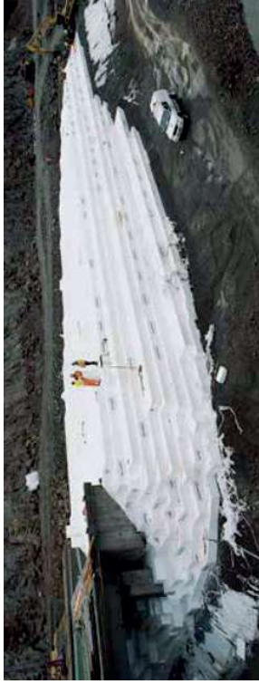
Figure 2.9 Geofoam block bridge approach embankment (Norway), (EUMEPS, 2010)
