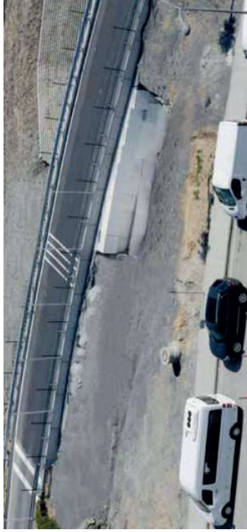
Figure 2.4 The use of both trapezoidal and vertical sides geofoam block configurations in the same project (Acıbadem – Üsküdar/Istanbul), (Özer & Akinay, 2017).
