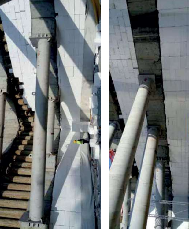
Figure 5.14. Geofoam block application in a deep excavation project (Place: Atakoy-Ikitelli Subway Bahariye Station, Bahariye-Ikitelli/Kucukcekmece, Istanbul, Date: 10.22.2018)
