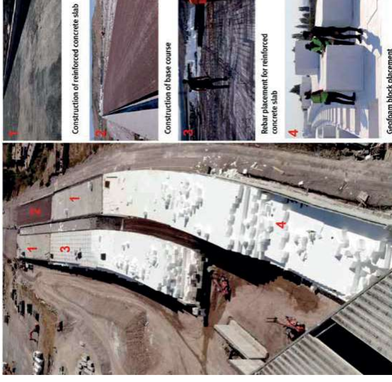
Figure 5.35 Simultaneous execution of the construction stages of geofoam bridge approach embankments (Place: Bogazkopru-Kocasinan/Kayseri, Date: 28.08.2019 – 15.10.2019)
